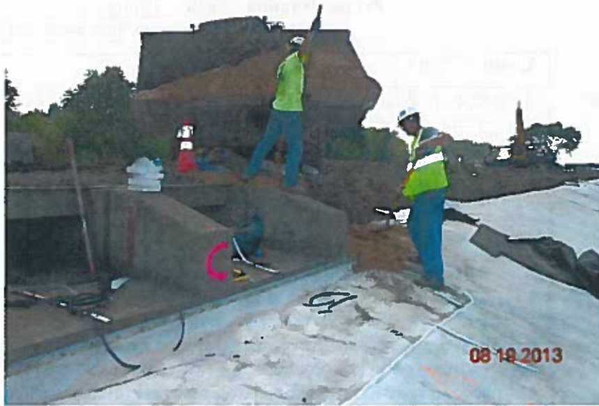
Placing sand around overflow structure (looking southeast)
