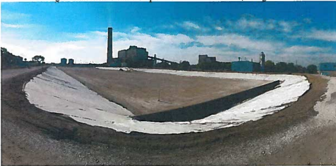
Panoramic view of entire basin from northeast corner, facing southwest
