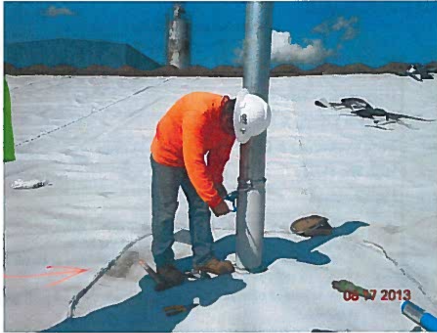
Geomembrane boot installation on a riser (looking west)
