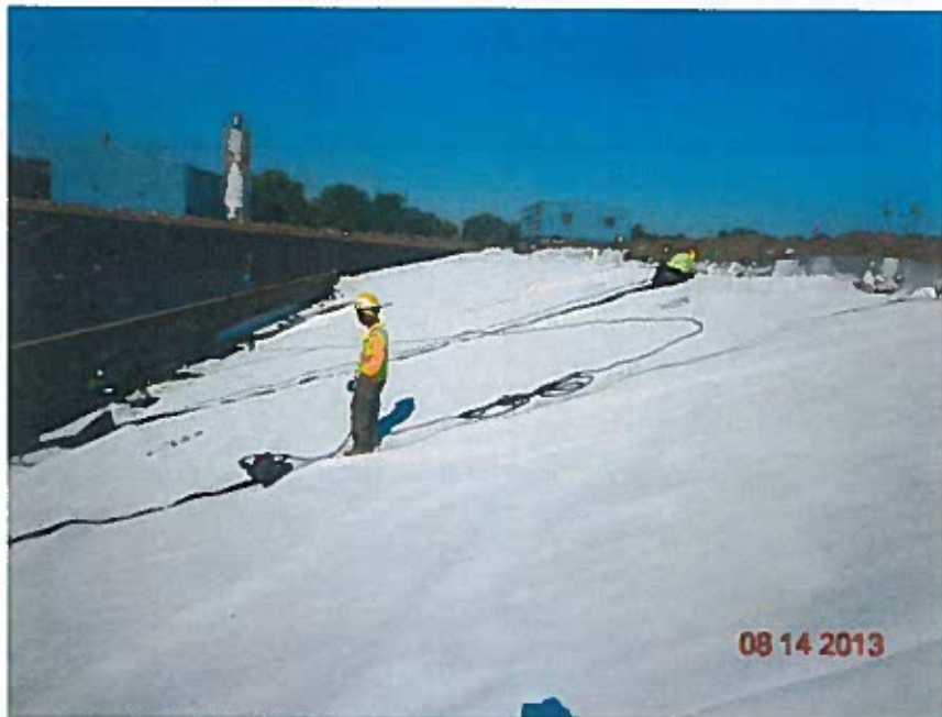
Seaming of the geomembrane panels (looking west)
