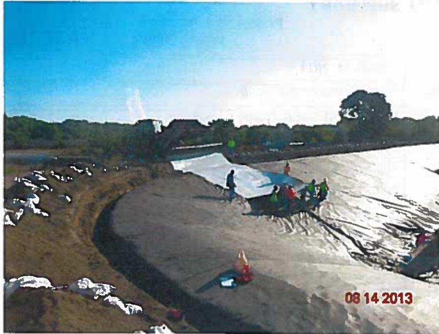
Rolling out the first HDPE Panel (looking northeast)
