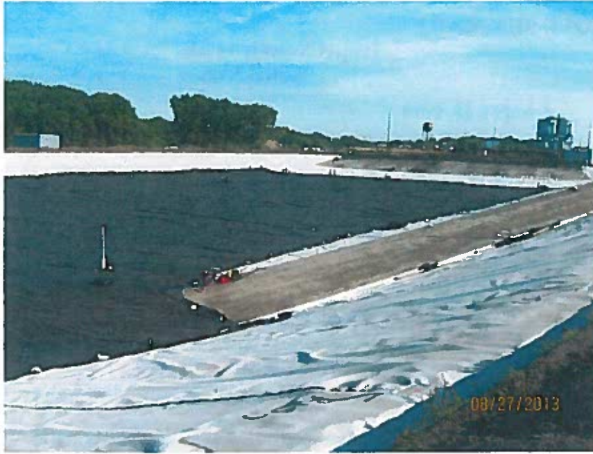
Extent of upper nonwoven geotextile installation completed to date (looking southeast)
