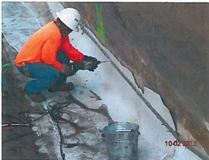
Repairs on batten strip
