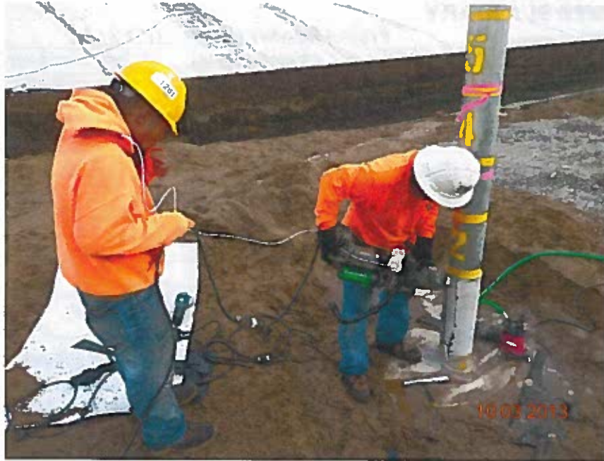
One of the riser pole geomembrane boots being fixed (looking north)
