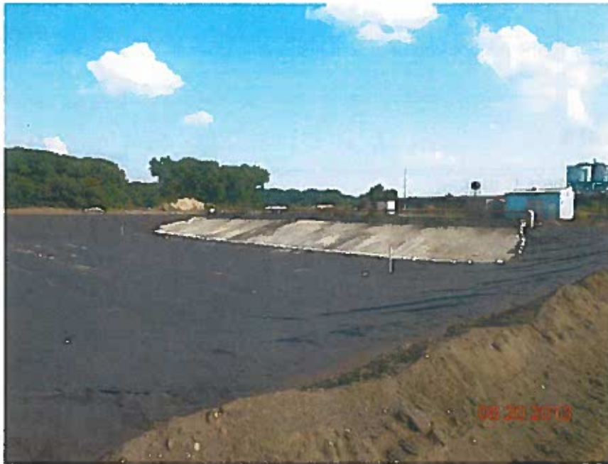
Extent of fabric deployment to the south (looking southeast)
