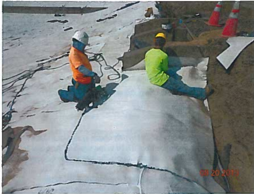
Second layer of geomembrane placed over clean, backfill sand (looking north)
