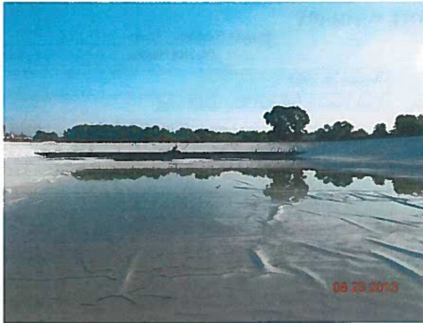
The flooded basin (looking north)
