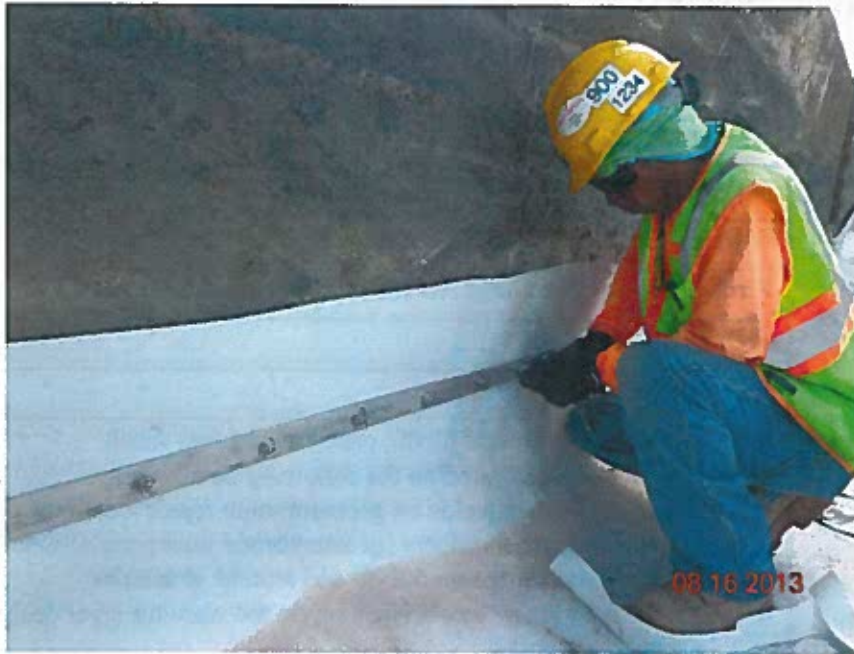
Batten strip connection along the outfall (looking south)
