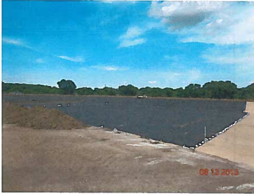
Extent of the day's nonwoven geotextile installation (looking northeast).
