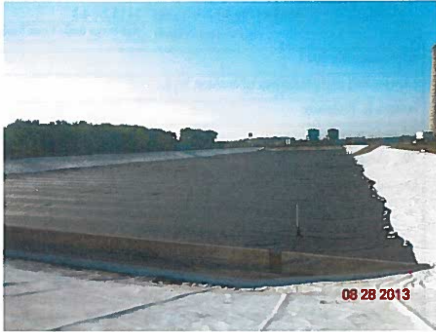
Extent of the completed geosynthetics (looking southeast)
