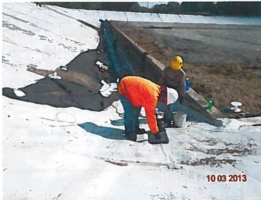
Vacuum testing a new patch along the weir wall (looking east)
