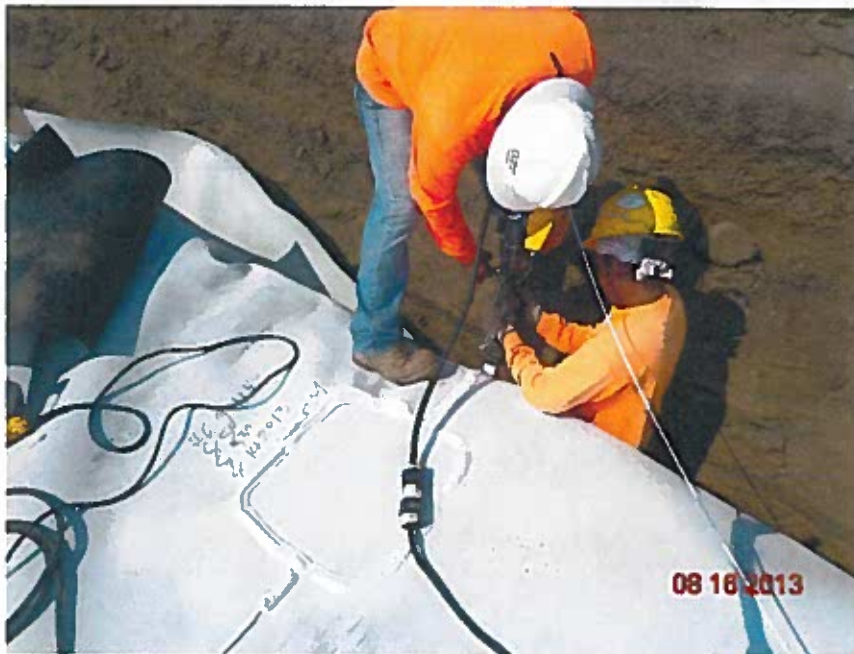
Extrusion weld on a repair location
