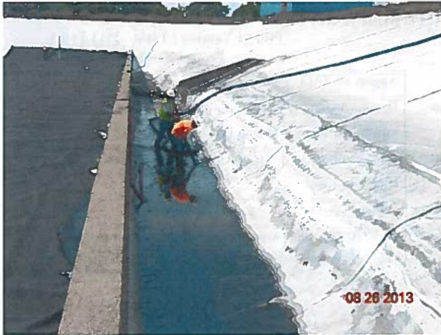
Dewatering the flooded basin (looking west)
