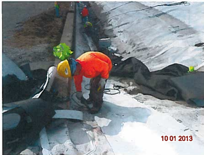
Batten strip repairs underway (looking west)
