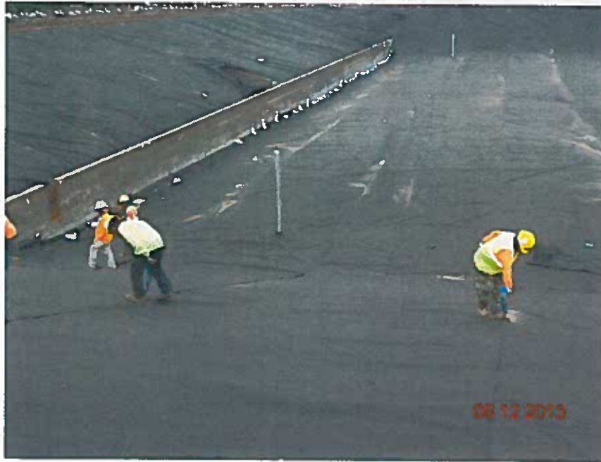
Heat bonding geotextile seams (looking east).
