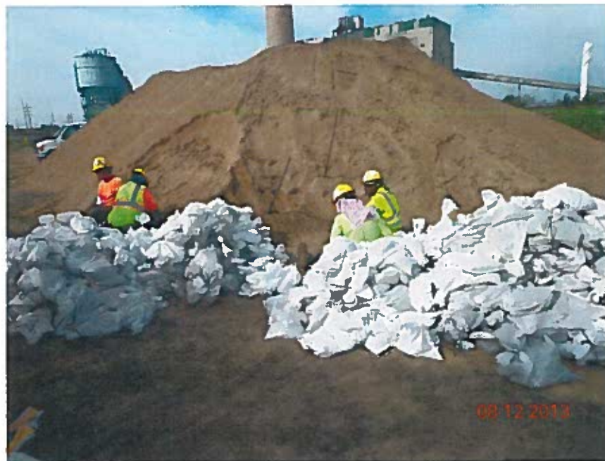
CAAWS crew filling sand bags ahead of the day's work.
