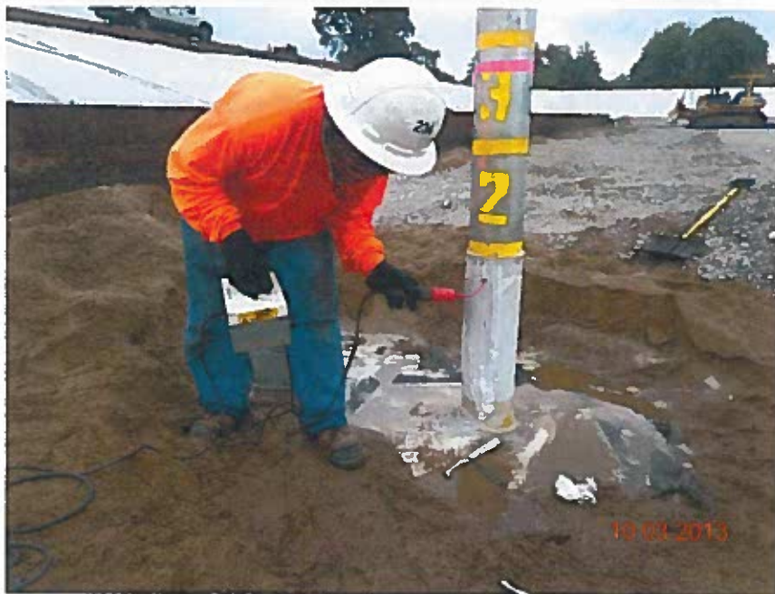
Spark testing the new repairs (looking northeast)
