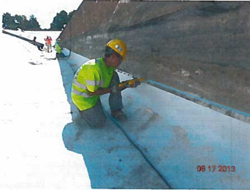
Caulking liner termination on the weir wall (looking east)
