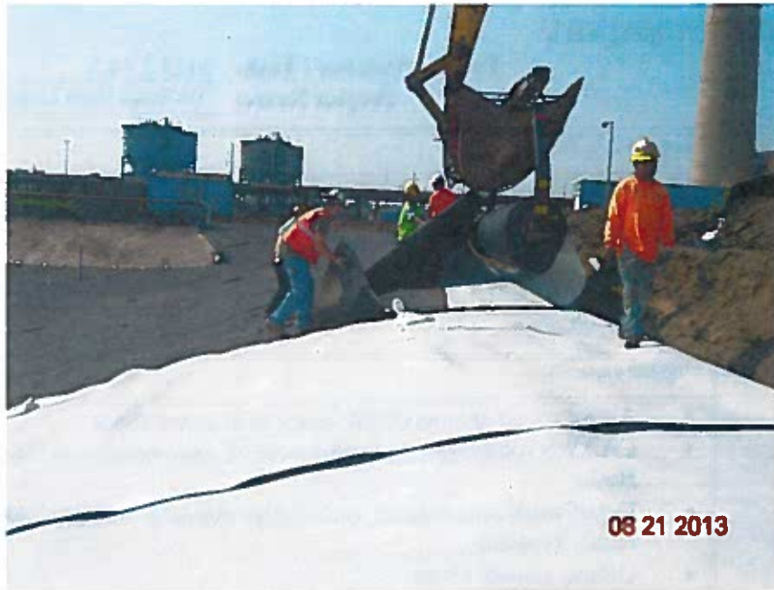
Geomembrane liner deployment towards the south of the basin (looking south)
