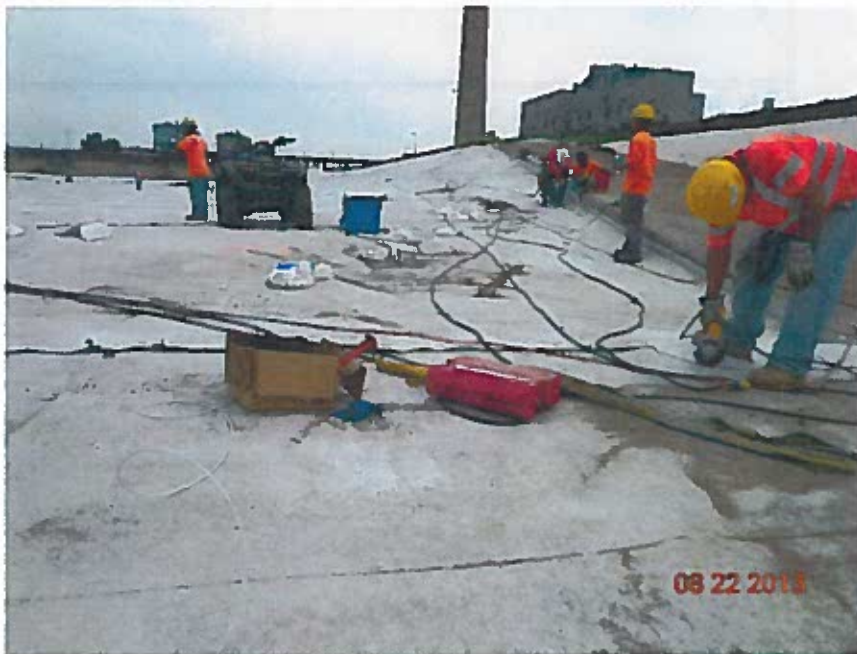
Repairing geomembrane along the ramp (looking southwest)
