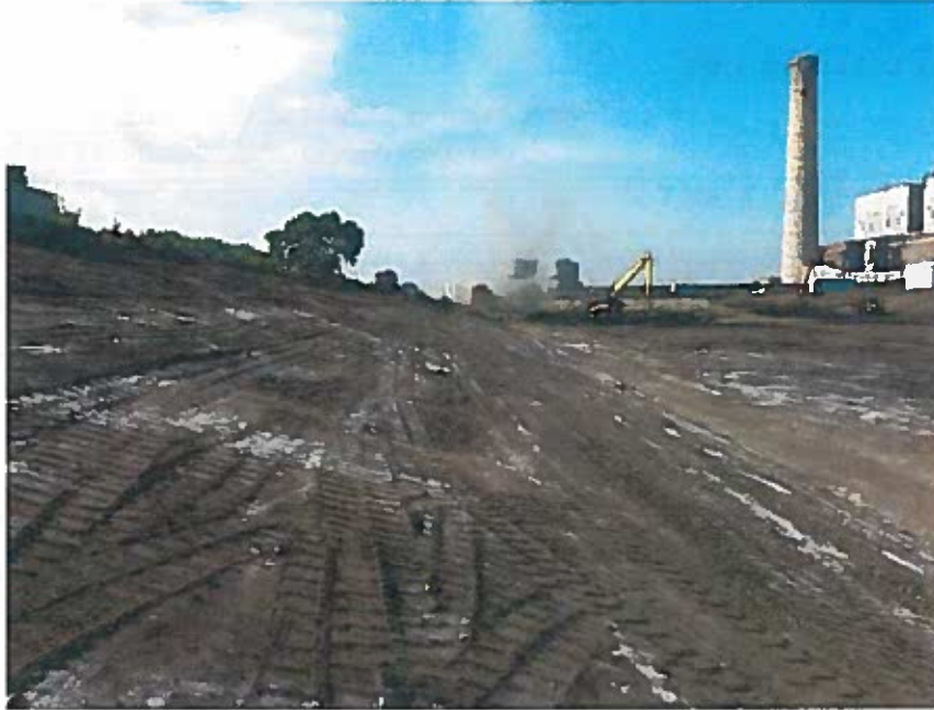
South-facing view of eastern slope, Poz-O-Pac and transition in good condition, some ash remains that will be removed
