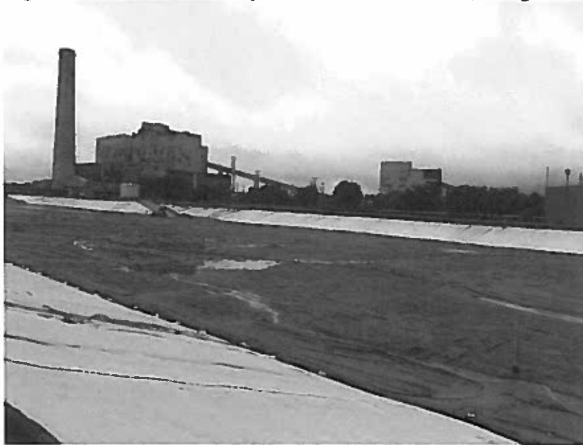
Dewatering basin after plug failure, facing southwest
