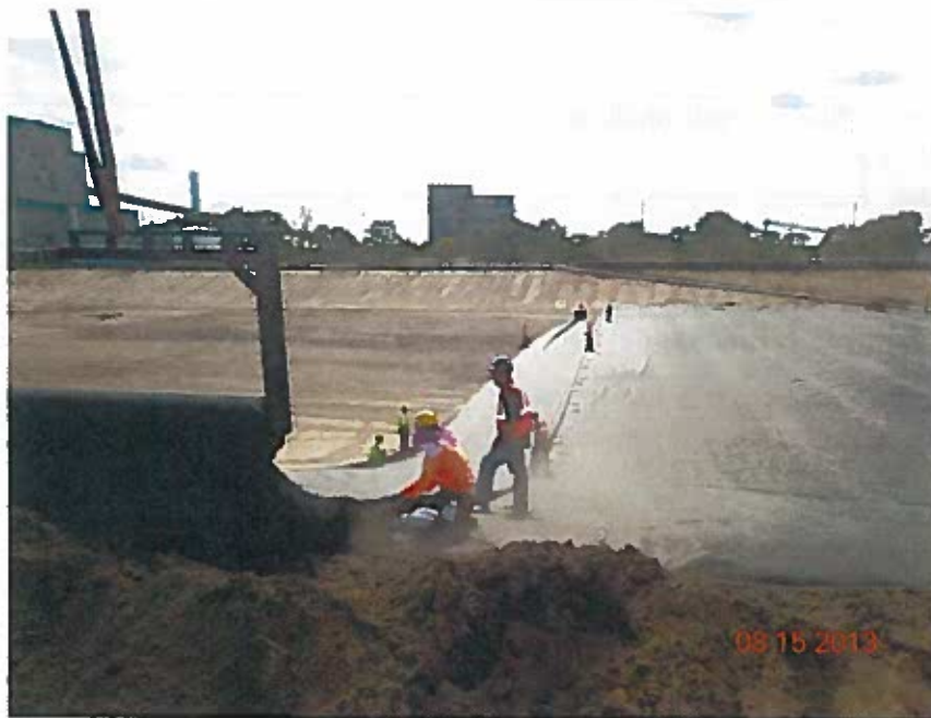
Deployment of geotextile (looking west)
