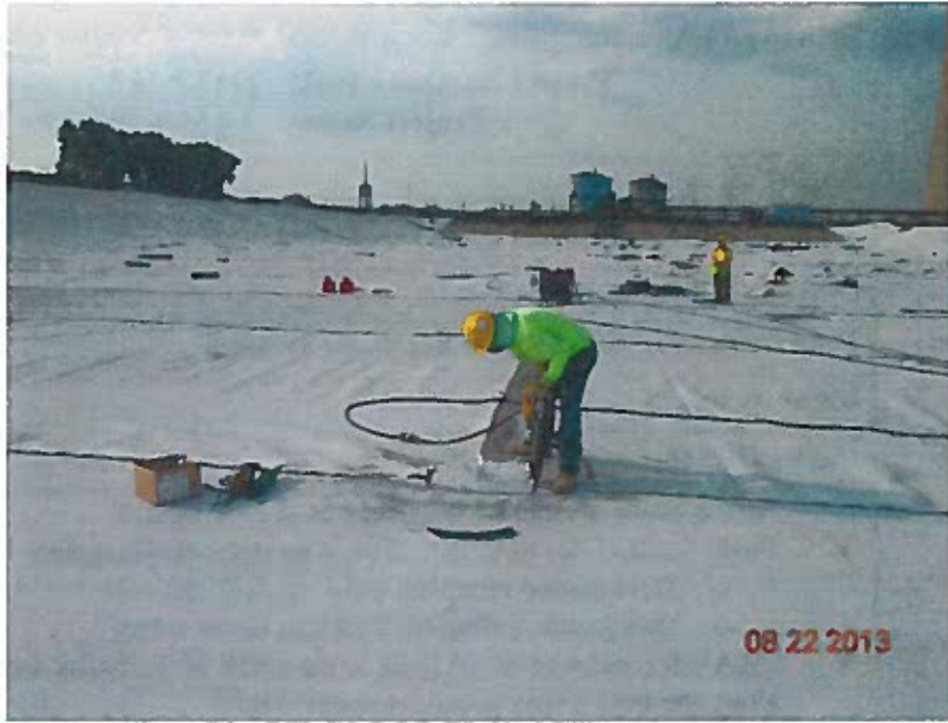
Extrusion welding a geomembrane repair in progress (looking south)
