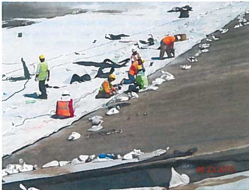
Geomembrane detail work along the inlet ramp (looking northeast)
