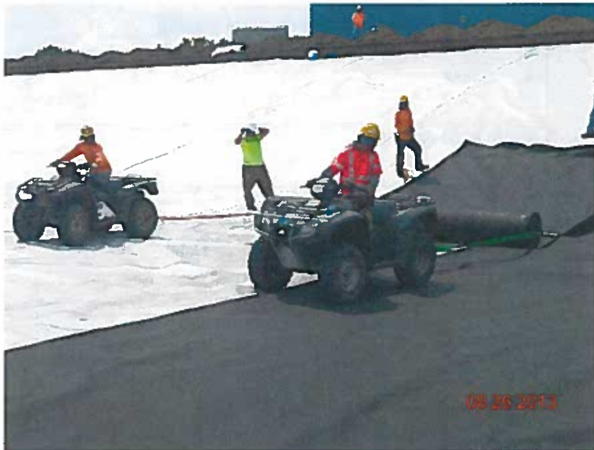
Deploying nonwoven geotextile fabric for the warning layer (looking southwest)
