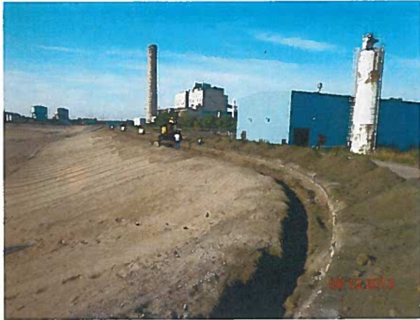
Terra Crew digging the anchor trench around the basin (looking southwest).
