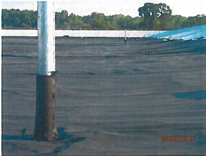
Geosynthetics liner penetration (looking north)
