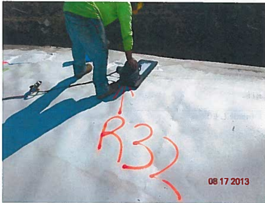
Vacuum testing a repair location
