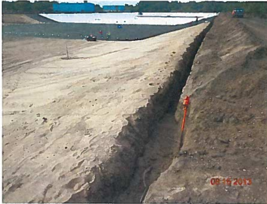
Extent of geotextile and HDPE deployment completed (looking north)
